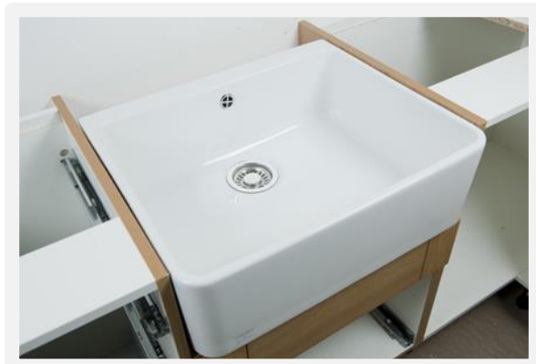
Position the sink and attach the waste.
